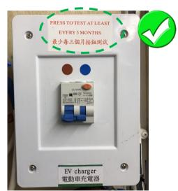
"最少每三個月按鈕測試" 及"Press to test at least quarterly"的告示應於電流式漏電 斷路器所在處或其附近提供。
